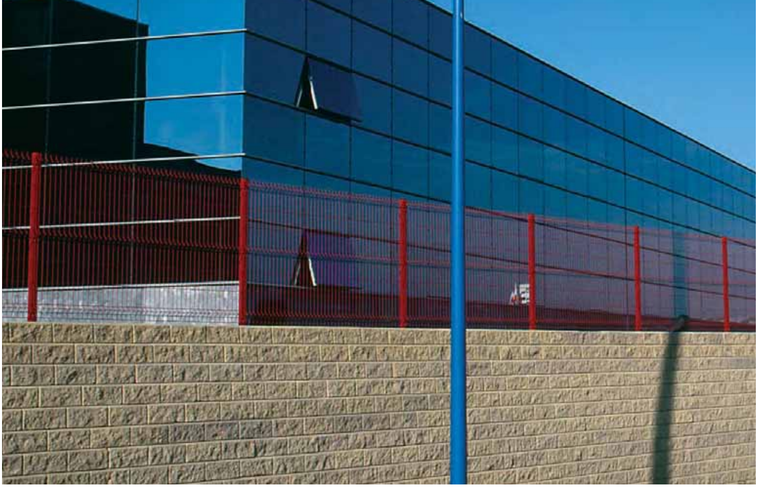
Industrial Estate "La Muela", Zaragoza. AB Three. Ref. Desierto
