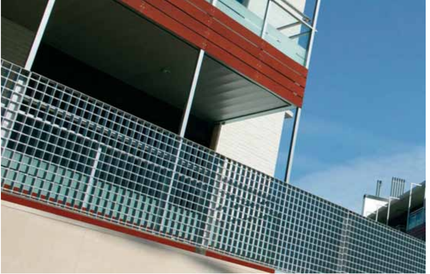
Block of flats in Tiana, Barcelona. Eduard Sabater. Hollow Brick. Ref. White Marble Construction project finalist in the private works category in the Maresme 2004 Triennial Architecture competition
