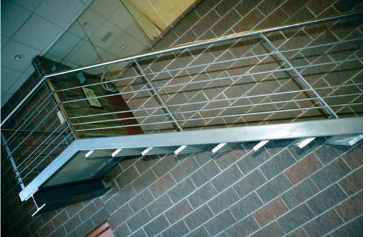
Office in Canovelles, Barcelona. Split face Block. Ref. Sierra / Oficinas en Canovelles, Barcelona. Bloque Split. Ref. Sierra
